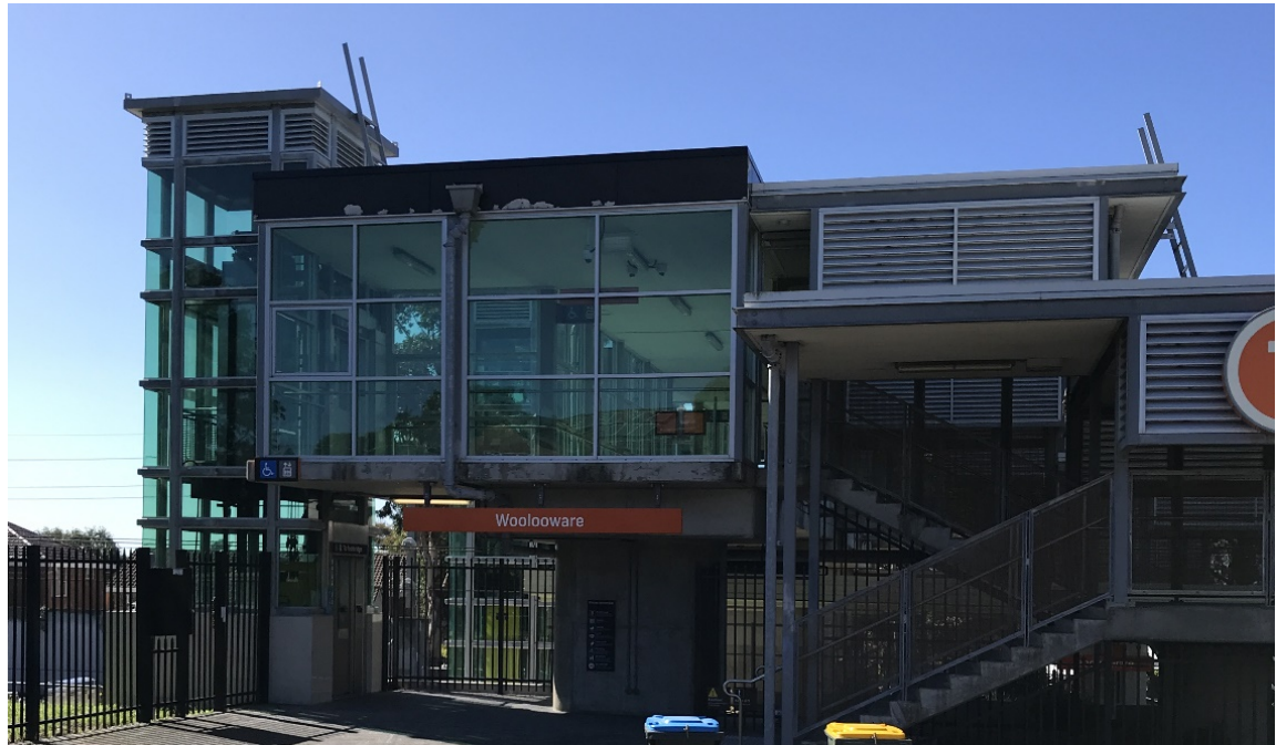
Photo P1: – View of Woollooware Station Entrance in Swan Street.
